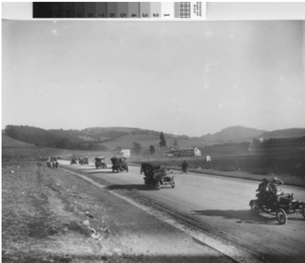
(Automobile Race on Foothill Blvd in Oakland----- 1909)
