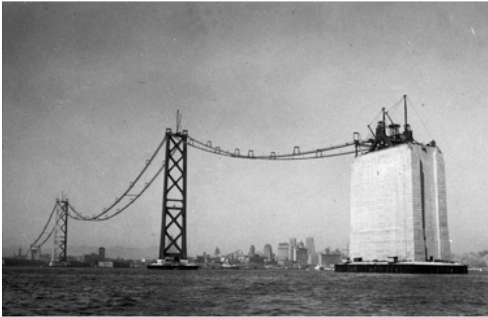
Construction of Oakland-Bay Bridge, 1933
